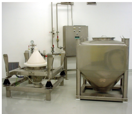
IBC & Discharge Station
