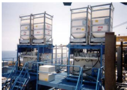
Offshore Filtration Operation
