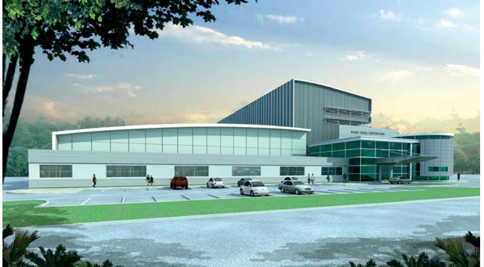
Seasoning and Freeze Dryer Facility
